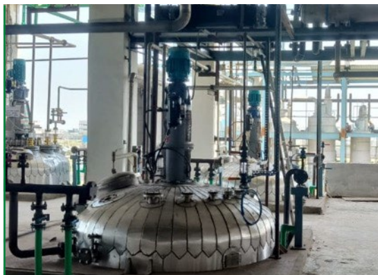
Reactor Installation Completed
