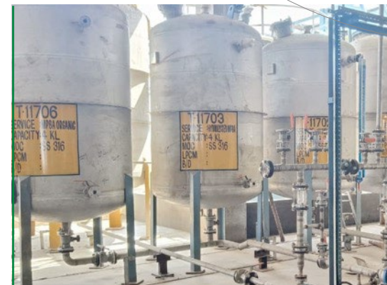
Reactor Installation Completed
