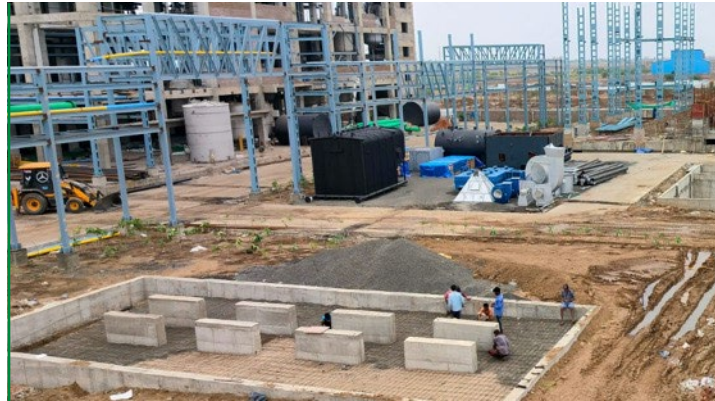
Foundation Works Completed of Isobutylene (RM) Tank
