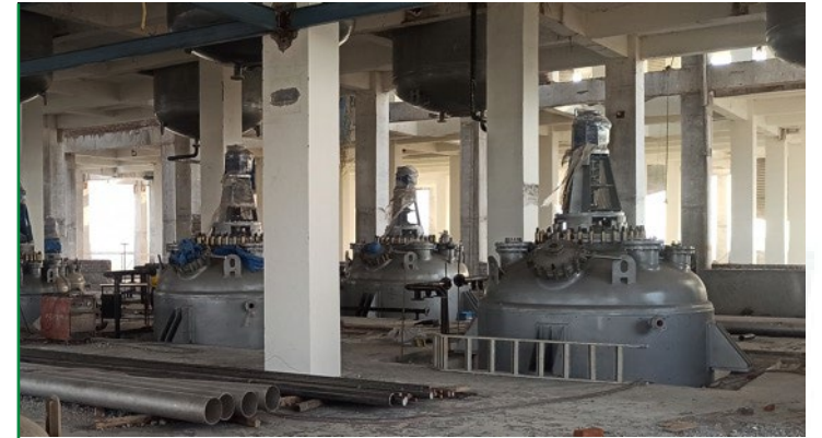
Reactor Installation
