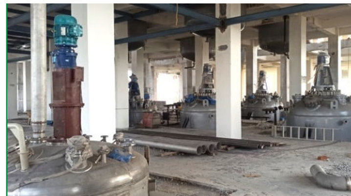
Reactors Installed & Piping Commenced
